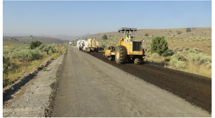
Compaction on Juntura Cutoff
