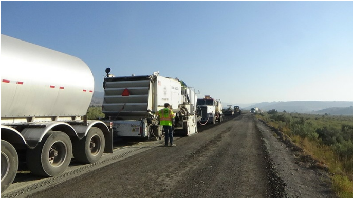
Juntura Cutoff with Portland Cement spread ready to be put in the mix
