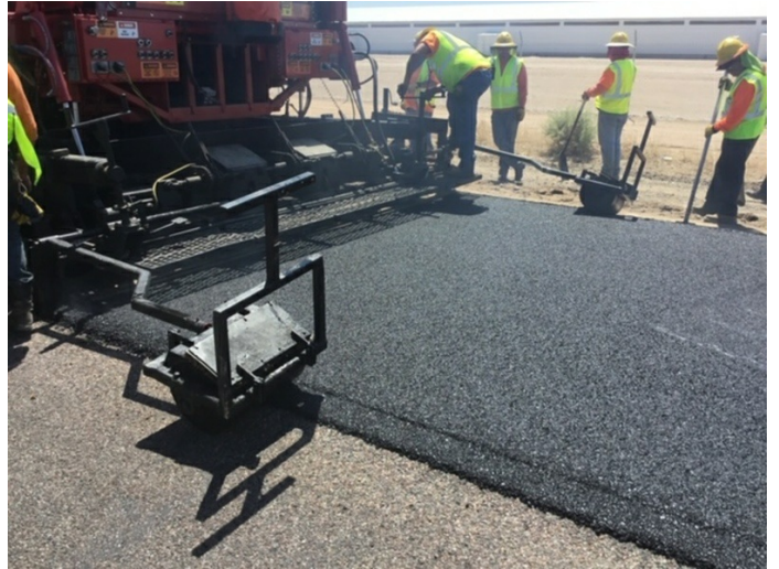
Final 1" recycled layer under 1" new layer AR.
