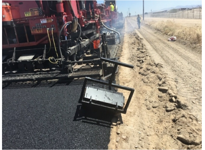
Hot in Place Repaving/safety edge
