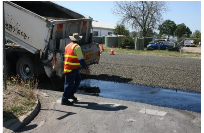
Installing the seal February 2014
