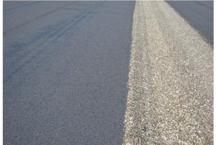
Installing the Micro Surfacing
