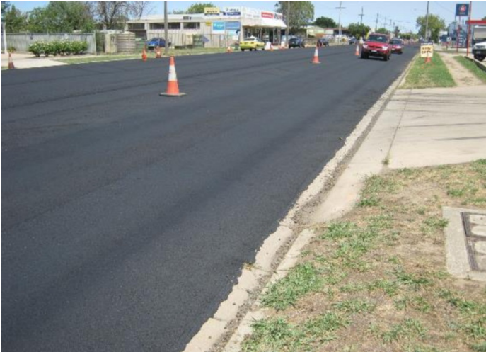
Installing the Micro Surfacing
