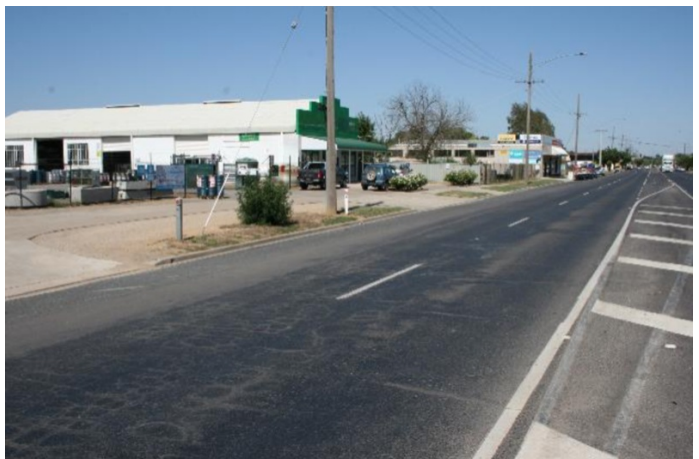
Pre-existing Condition - January 2014
