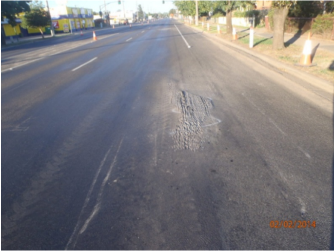
Pre-existing Condition - January 2014
