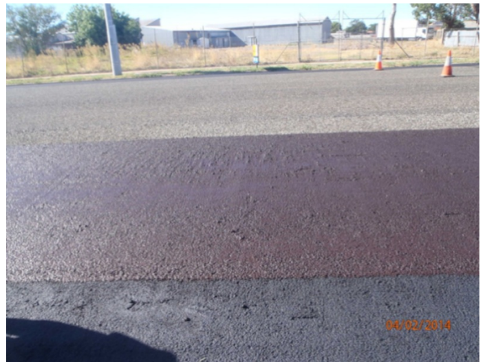
Installing the Micro Surfacing
