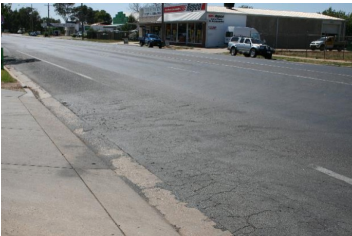
Pre-existing Condition - January 2014
