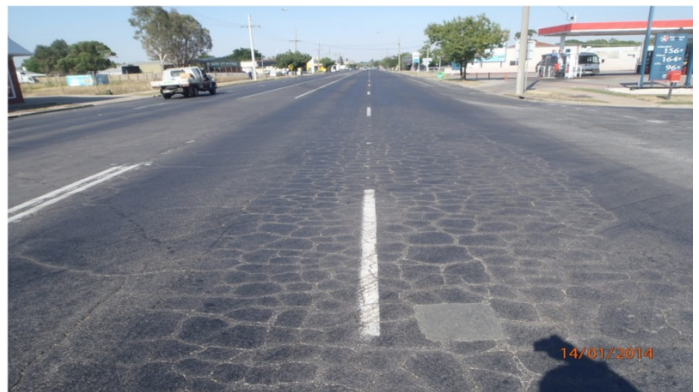
Pre-existing Condition - January 2014
