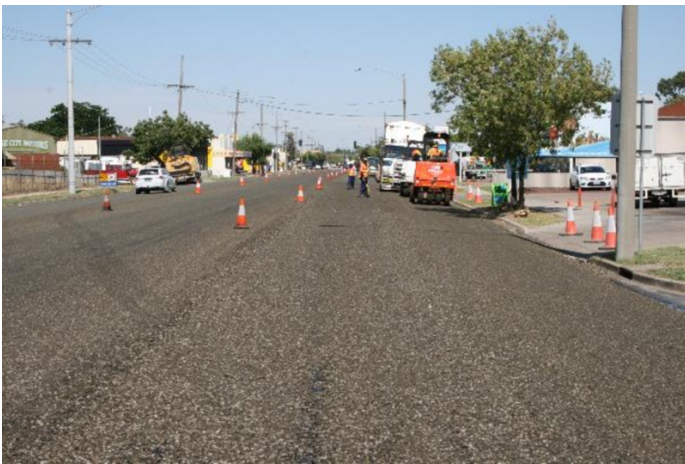
Installing the seal February 2014
