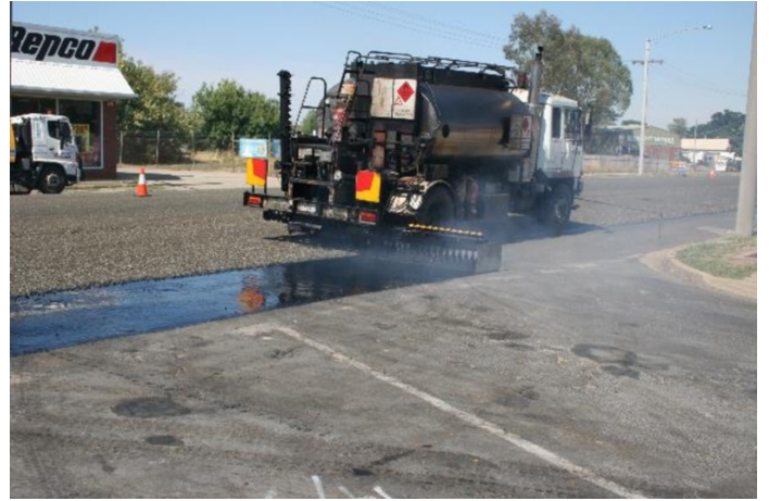
Installing the seal February 2014
