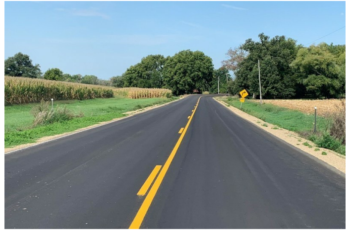
Finished Project with Cape Seal Surface
