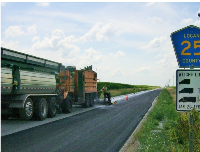
Applying the Microsurfacing
