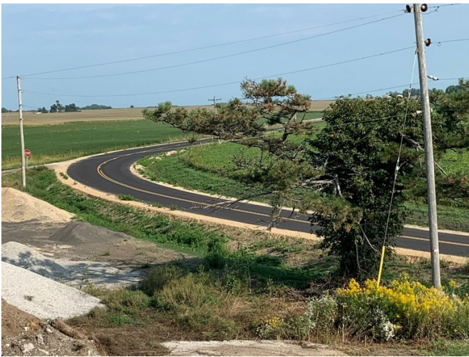
Safety Enhanced in Curves with FDR and Widening
