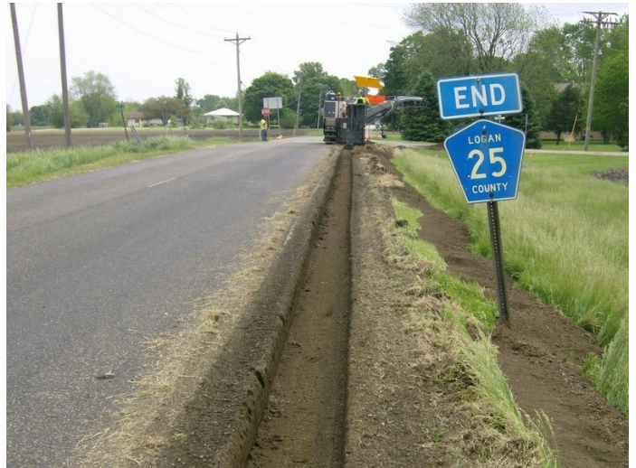
Trenching Material for Widening with FDR
