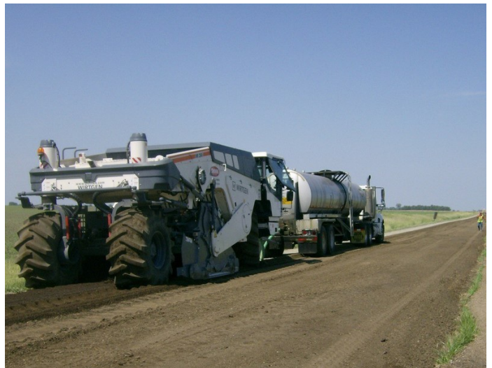
FDR Stabilization with Engineered Asphalt Emulsion
