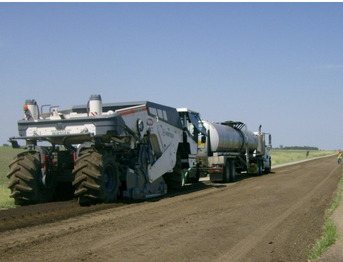
FDR Stabilization with Engineered Asphalt Emulsion
