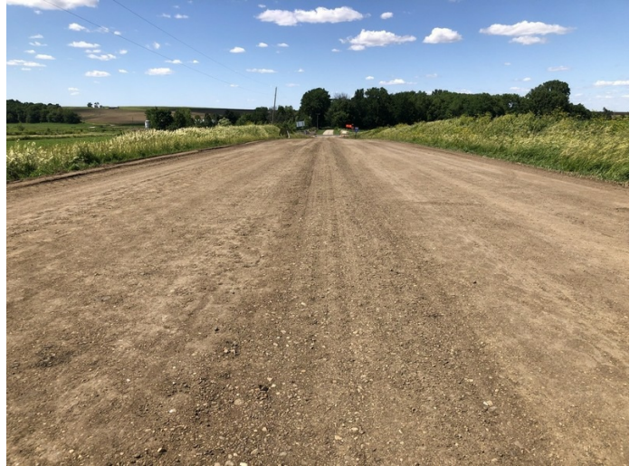
Finished FDR mat
