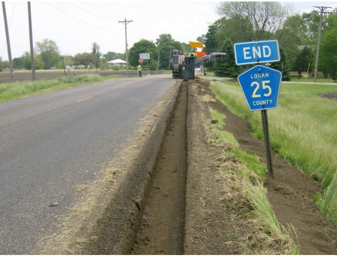
Trenching Material for Widening with FDR
