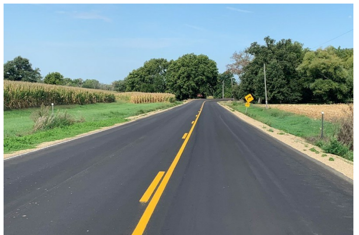
Finished Project with Cape Seal Surface
