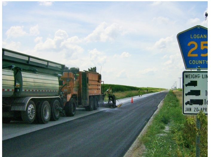
Applying the Microsurfacing
