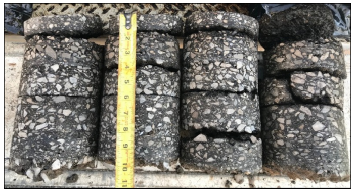
Pavement Samples taken during Investigative Sampling
