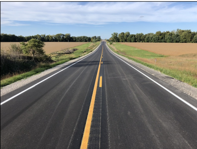
Final pavement surface
