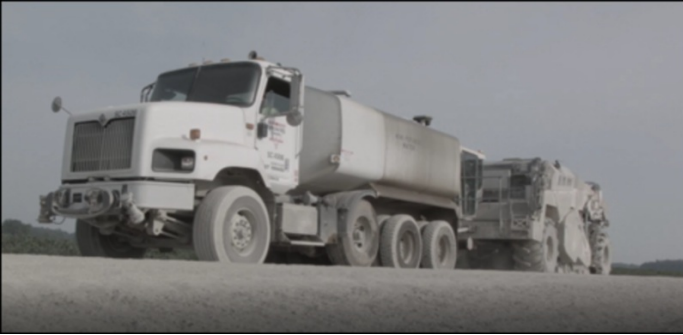
10.0-inch Cement FDR process
