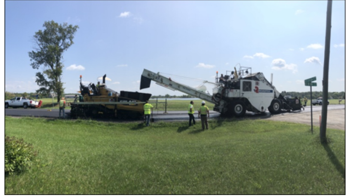
Paving of the 2.0-inch 12.5mm HMA surface
