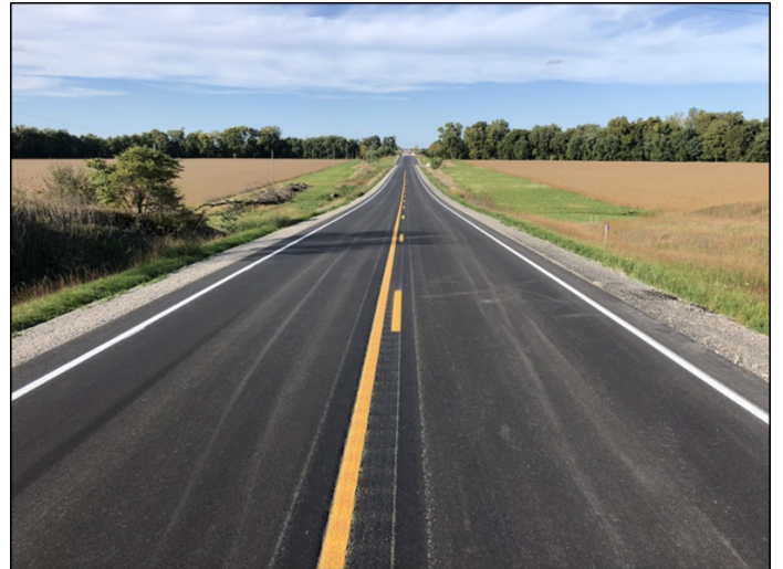
Final Pavement Surface
