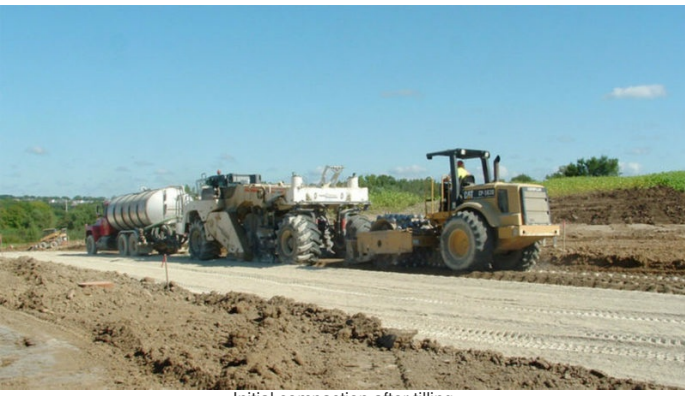
Initial compaction after tilling
