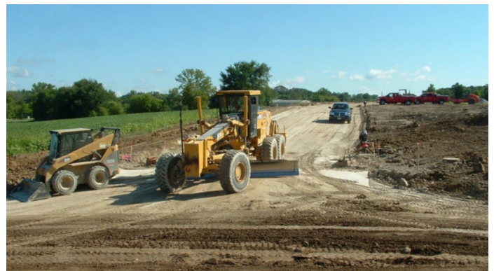
Final grading to elevation
