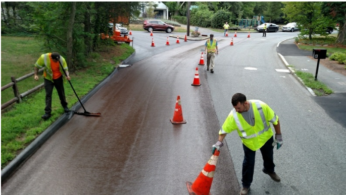
View from Operator's Platform
