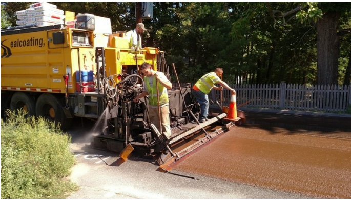
Application of Microsurfacing
