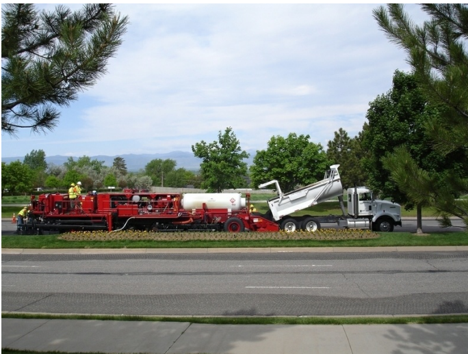
Cutler Repaving's single pass recycling process completes the recycling and resurfacing simultaneously, thereby minimizing delay and inconvenience to the traveling public.
