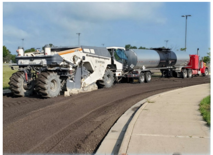
Performing FDR with emulsified asphalt
