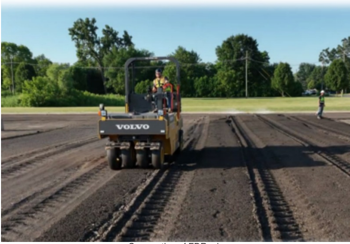
Compaction of FDR mix
