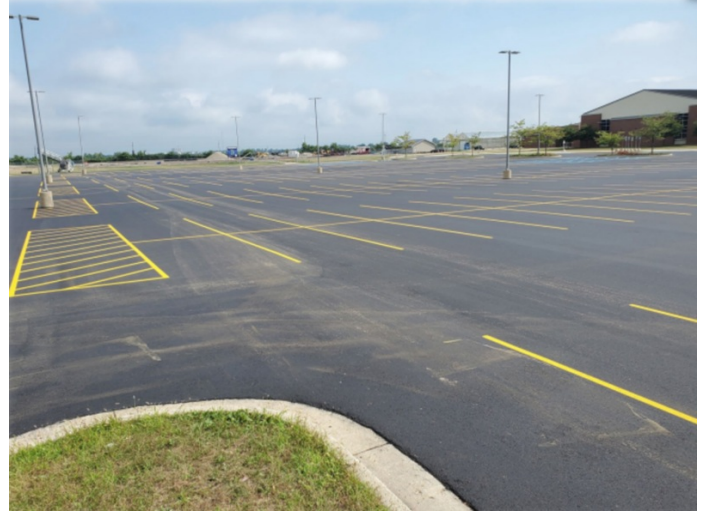
Completed parking lot
