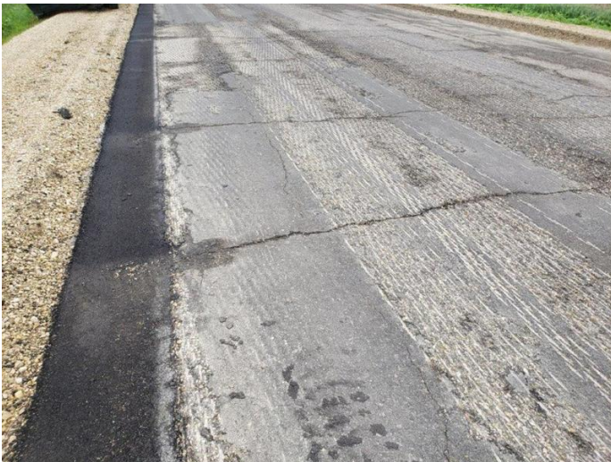
Sinclair Ave after profile milling
