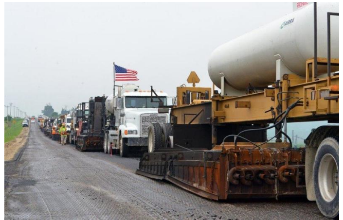
Performing 2-inch HIR on Sinclair Ave
