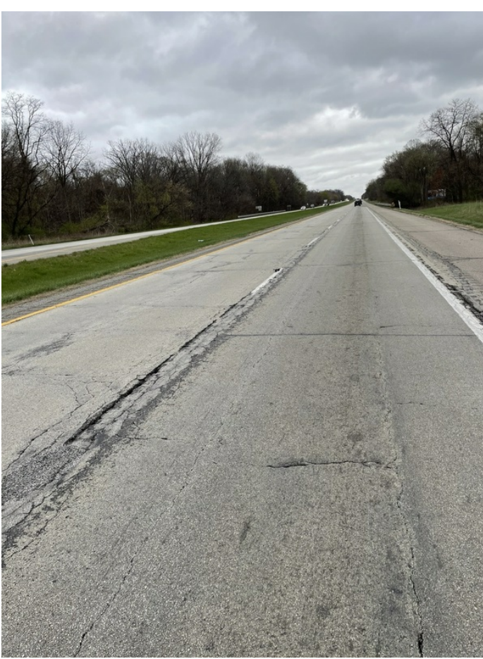
Existing Pavement Surface during Investigative Sampling
