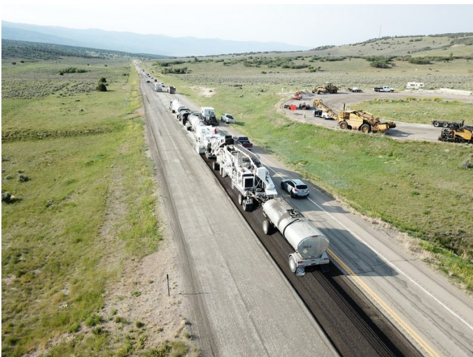
Coughlin Company Multi-Unit Cold In-Place Recycling train in the cut on US 89
