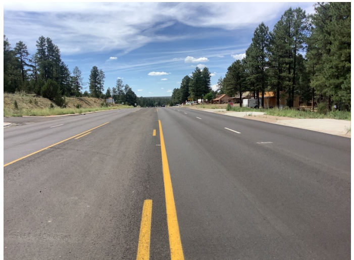
Completed project on SR-260 in Arizona
