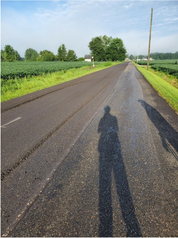
Compacted and uncompacted CIR mat on Jackson Road
