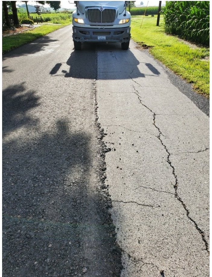
The compacted 5.0-inch CIR mat next to the distressed existing pavement
