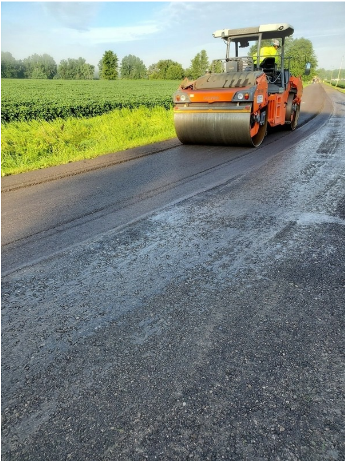
The smooth drum roller compacting the CIR mat
