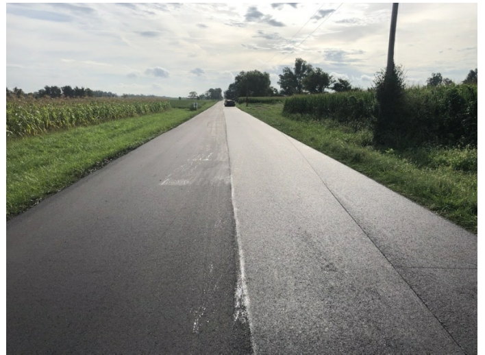
Finished 1.5-inch HMA surface on Jackson Road
