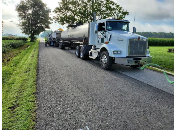
The Multi-Unit train processing Jackson Road
